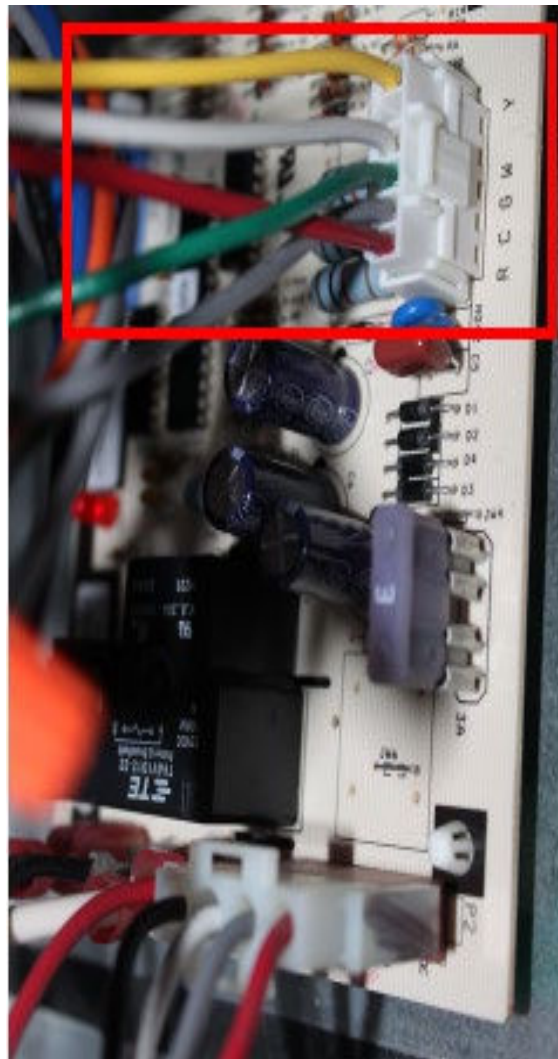
Figure 6: HVAC Equipment Control Board Connection Plug Field connections wire nut to wires (not shown)
